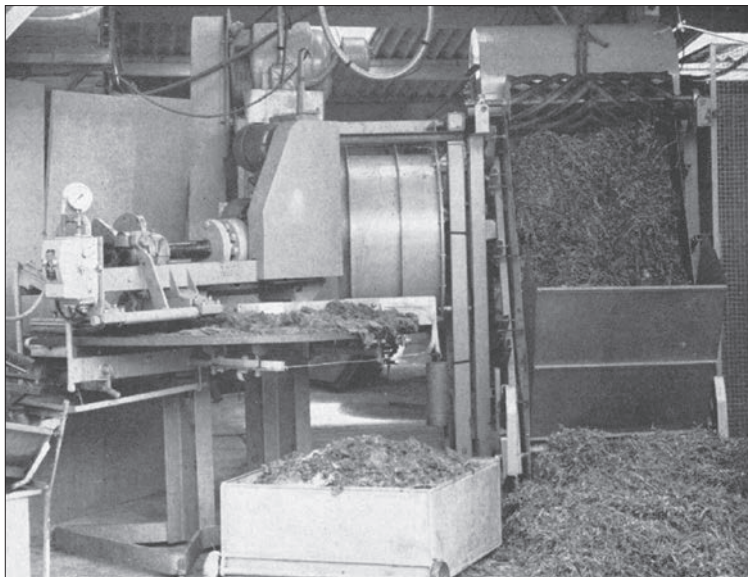
Photograph 1. Pilot machine used by N. W. Pirie for wet fractionation of green alfalfa (after Pirie, 1961)
